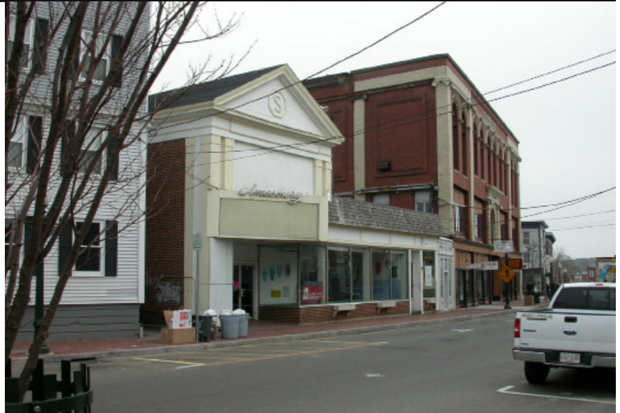
EXISTING FACADE - BEFORE RENOVATION
