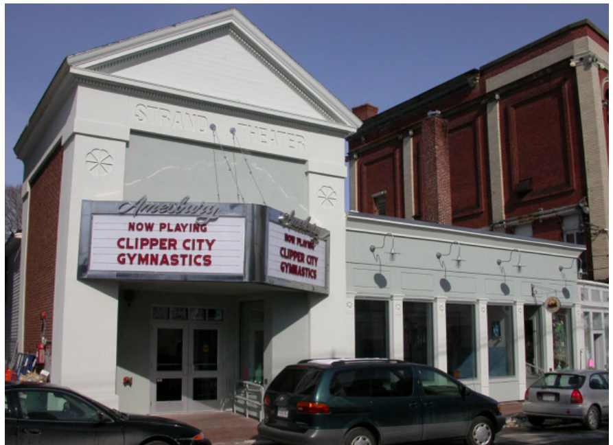
NEW FACADE - COMPLETED 2005
